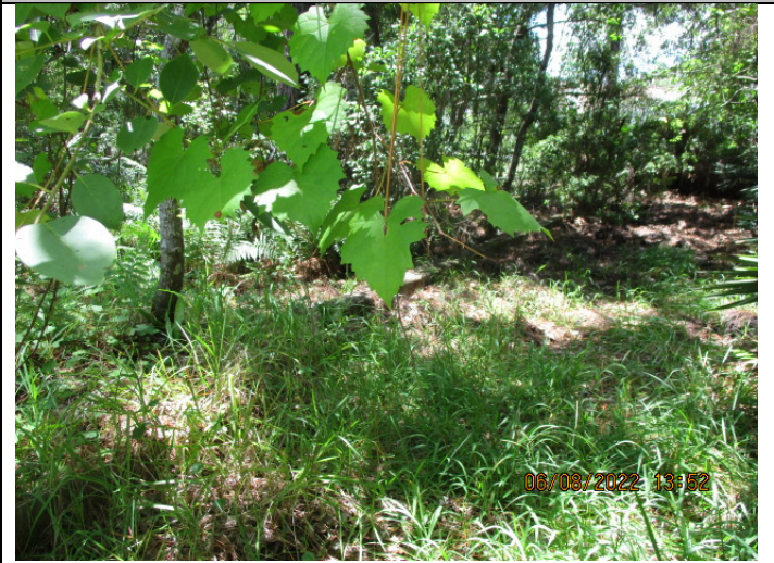
Image 6: Weir, Skimmer barely visible, needs clearing both sides
