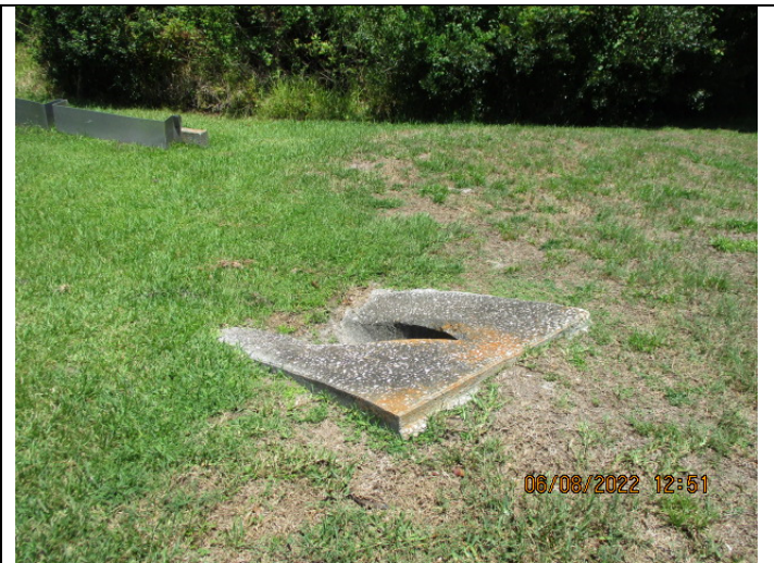
Image 2: MES/Pipe discharges towards Weir, swale may need minor exaction
