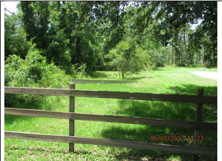
Image 8: Weir, Skimmer, needs minor clearing
