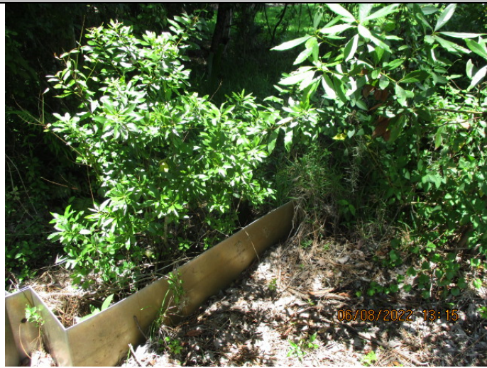
Image 3: Weir, Skimmer, needs clearing
