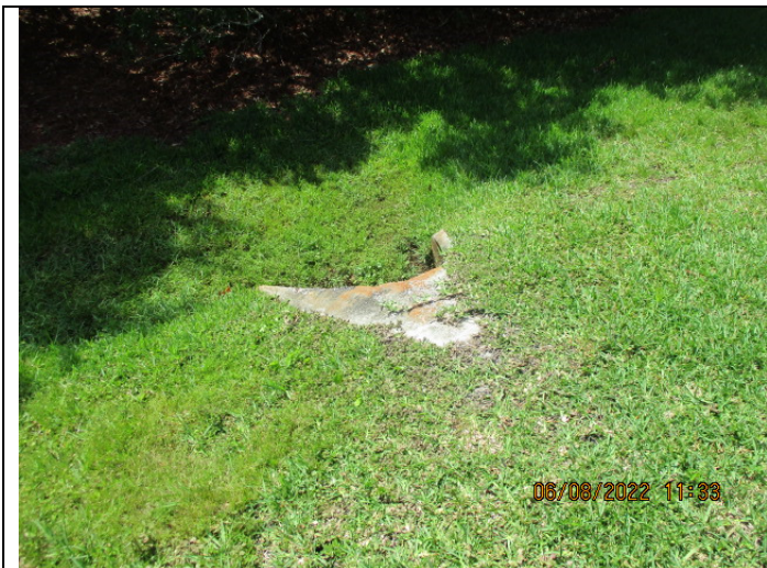
Image 1: FES/Pipe inlet connects road swale to swale that discharges to wetland
