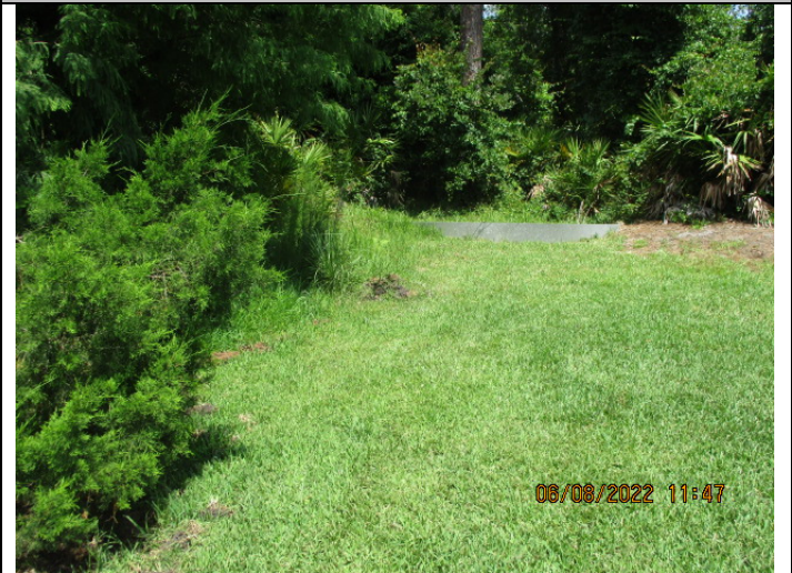
Image 10: Weir Structure at wetland discharge area
