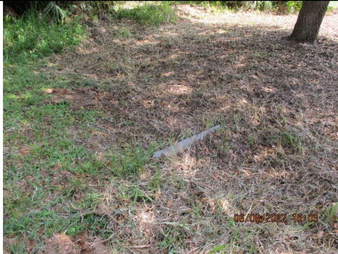
Image 3: Weir, skimmer needs clearing, re-cut swale
