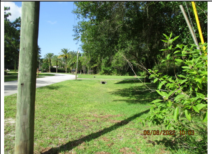
Image 12 : Front Swale along road, Ok
