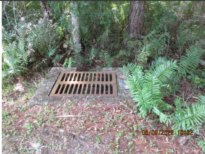
Image 5: Inlet basin connects to pipe system that connect wetlands
