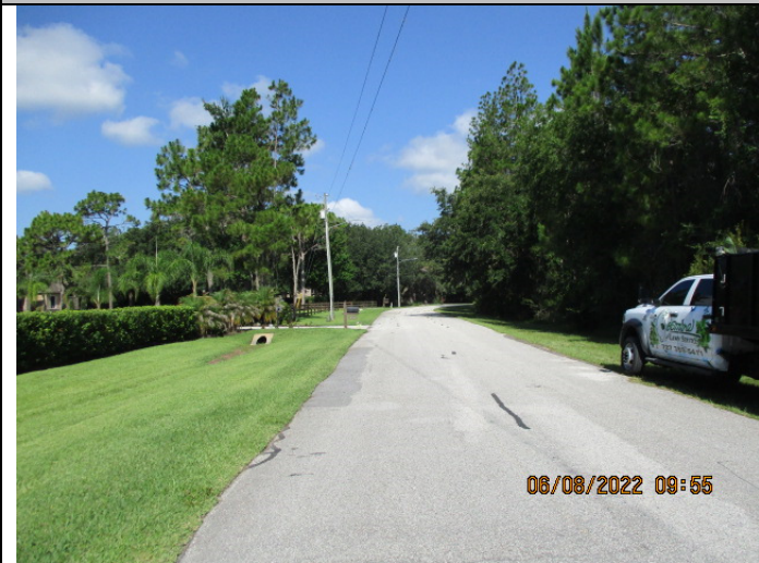
Image 11: Front Swale along road, Ok
